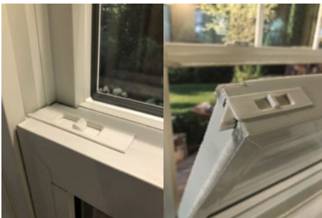
Tilt latches to make window cleaning easy!
